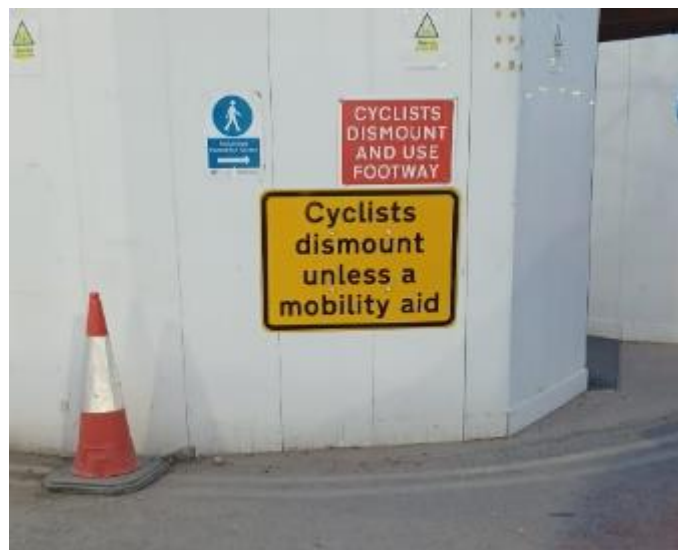
16. Works signs enabling inclusive cycling at Boord Street Bridge, Greenwich, 2023
