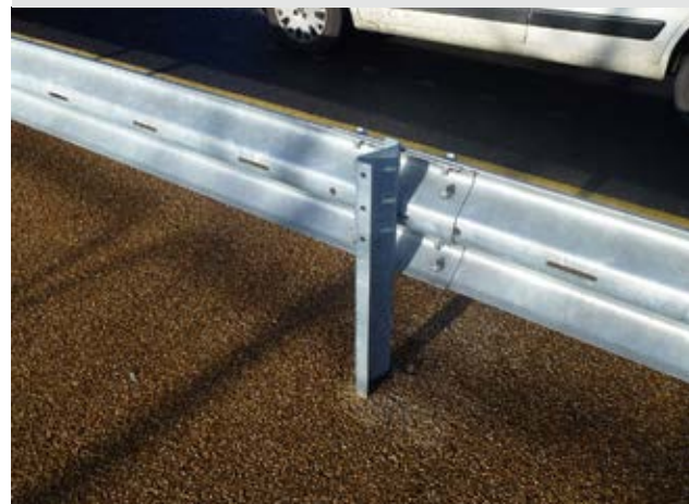
Figure 256: Barrier provision is essential on certain roads across the network
