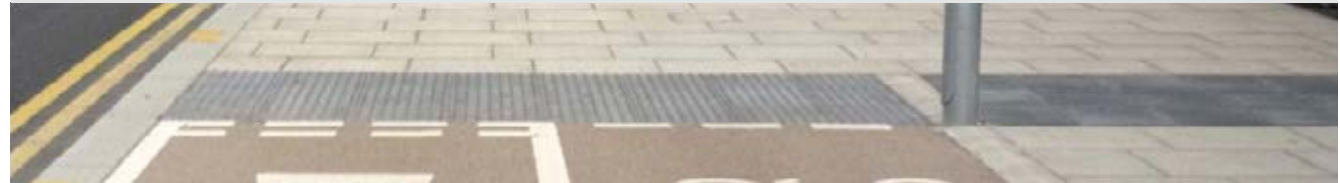
Figure 134: Ladder and tramline paving 800mm width on Borough Road
