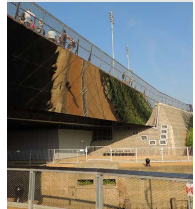
Figure 160: A footbridge in Queen Elizabeth Olympic Park in Stratford, London
