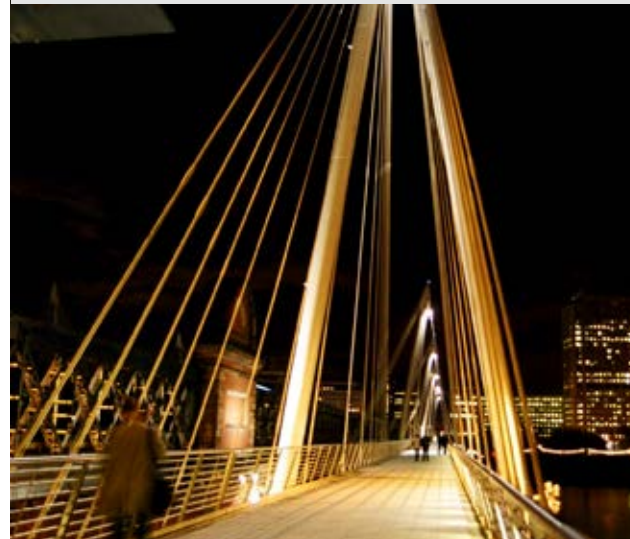
Figure 167: One of the Golden Jubilee footbridges
