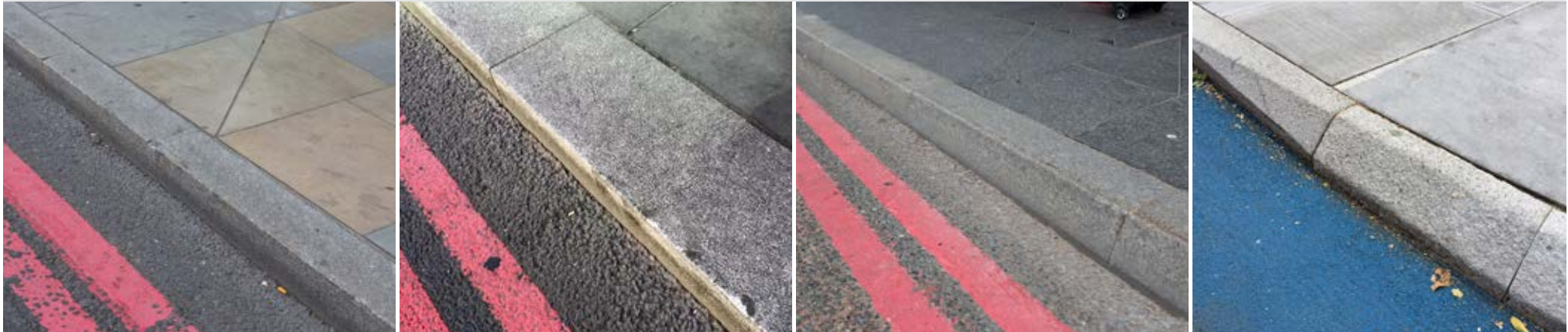
Figure 95: A selection of kerbs on the TLRN
