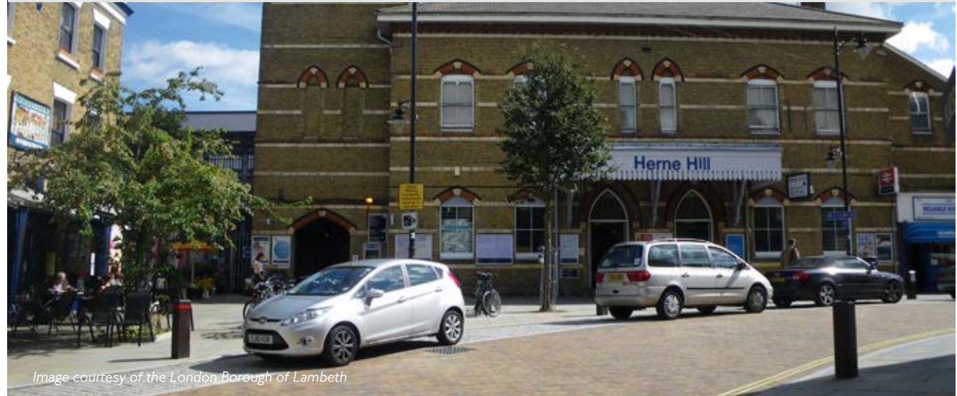
Figure 22: Strong relationships and flexibility throughout the design process has led to a multifaceted and vibrant space which is actively used by the local community and provides a distinct sense of arrival at Herne Hill
