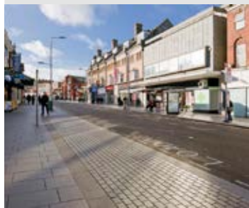
On footway – flush kerb
