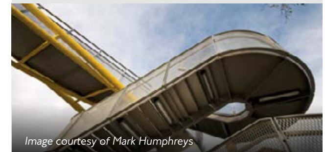
Figure 169: Necessary structural elements can be designed to be beautiful elements in their own right
