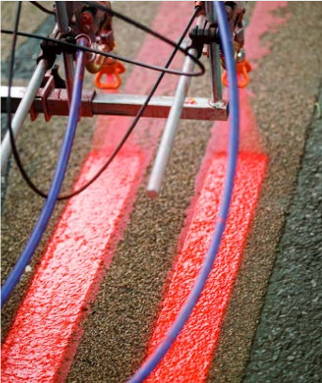
Figure 108: Renewed red line markings
