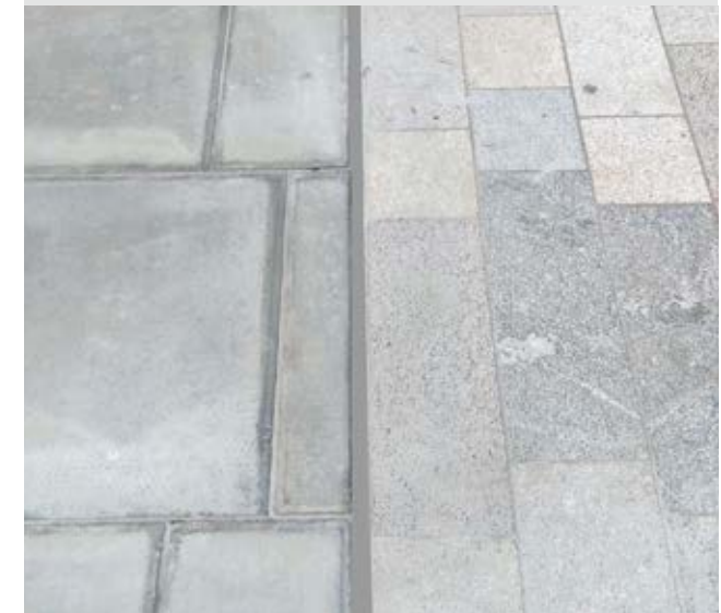
Figure 76: 900x600mm concrete slabs transitioning to granite
