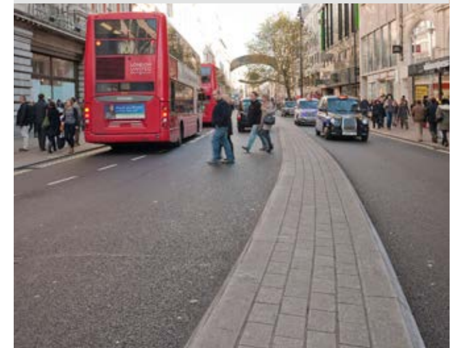
Figure 122: Oxford street's central median is paved in granite setts to match the concrete paving on the footways
