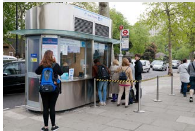
Figure 309: River pier ticket kiosk
